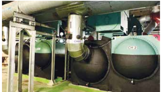
Chiller replacement at MVM
